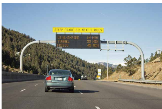
Real-Time Traffic Status Display
