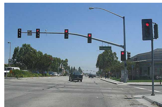
Traffic Signal Control
